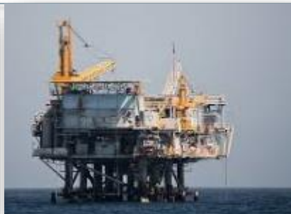
Topside, jacket and dropped object inspections.
