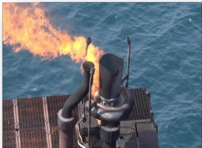
Live offshore and onshore flare inspections.
