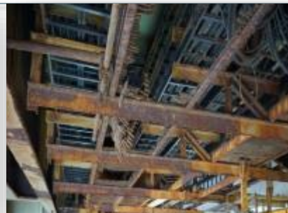
Under deck and splash zone.
