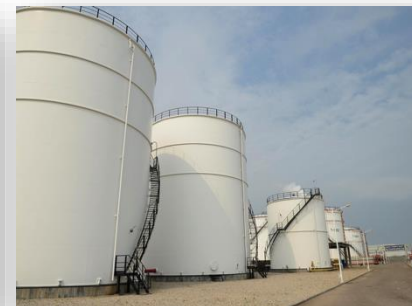
Storage tanks and silos (internal / external)
