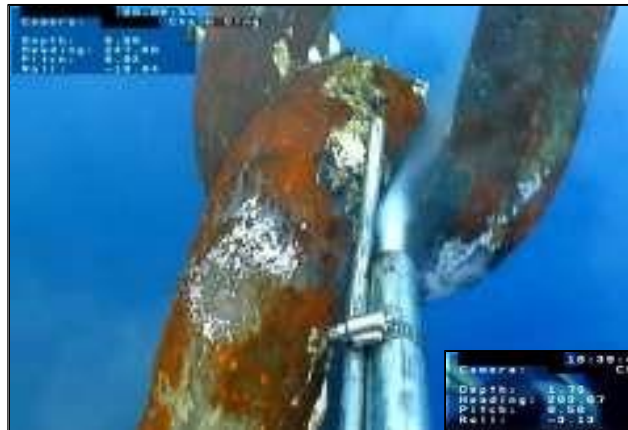
Spot Cleaning of Mooring Chain Prior to Thickness Measurements
