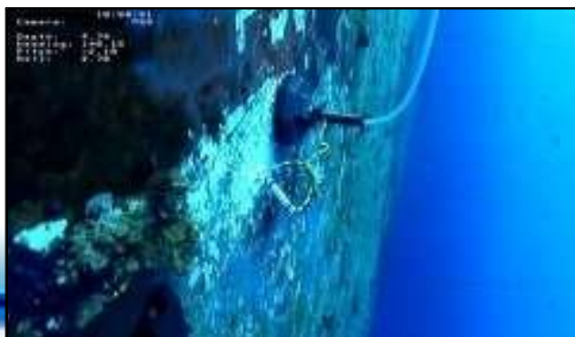
Sea-valve successfully plugged
