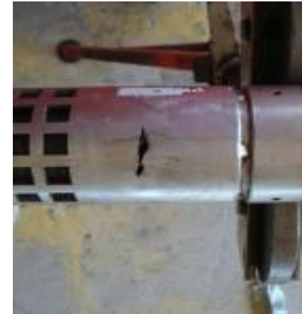
Erosion at box Module #3
